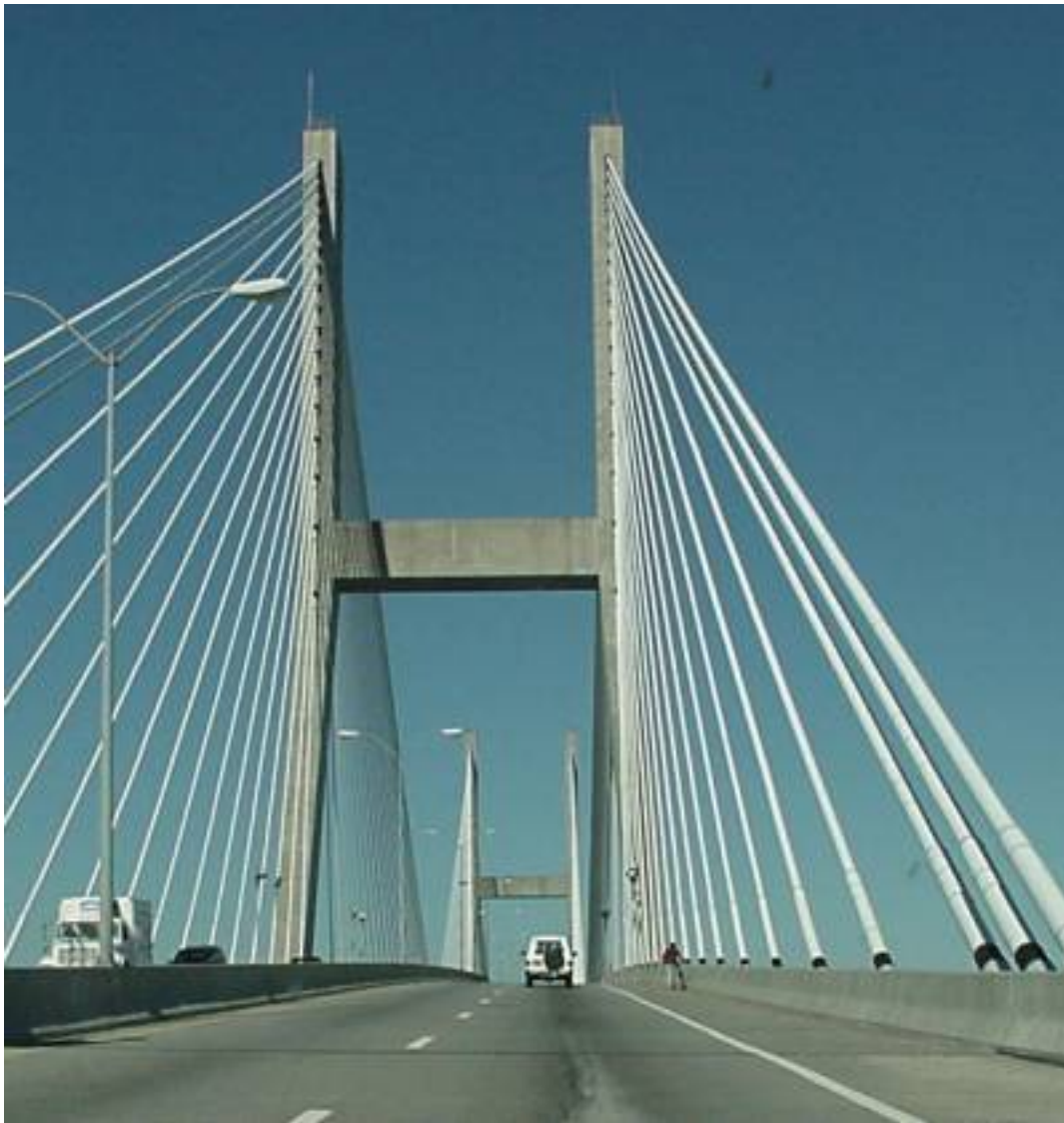
A cable-stayed bridge near Savannah, Georgia, USA
